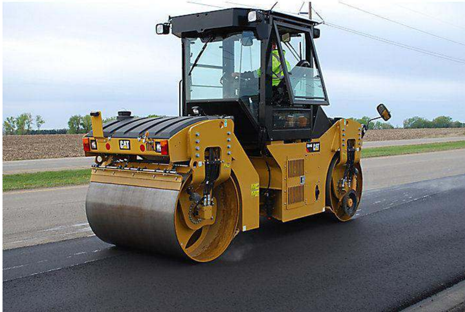
Gambar 6.26 Pengoperasian Tandem Vibratory Roller
